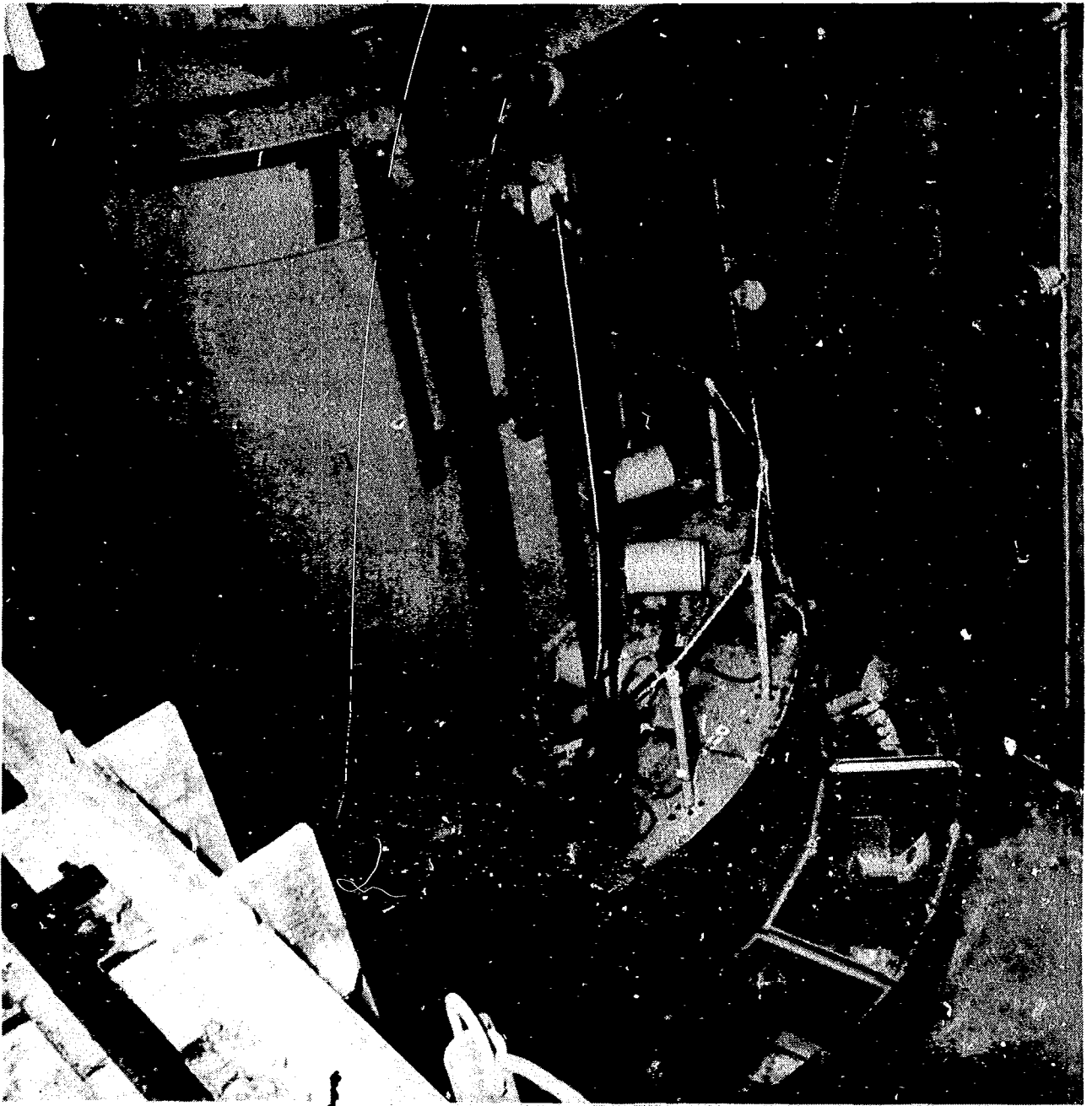
Figure 7. Service structure showing fans and exhaust ports, neutron shield tanks, walkway over reflective insulation, and hoist.
