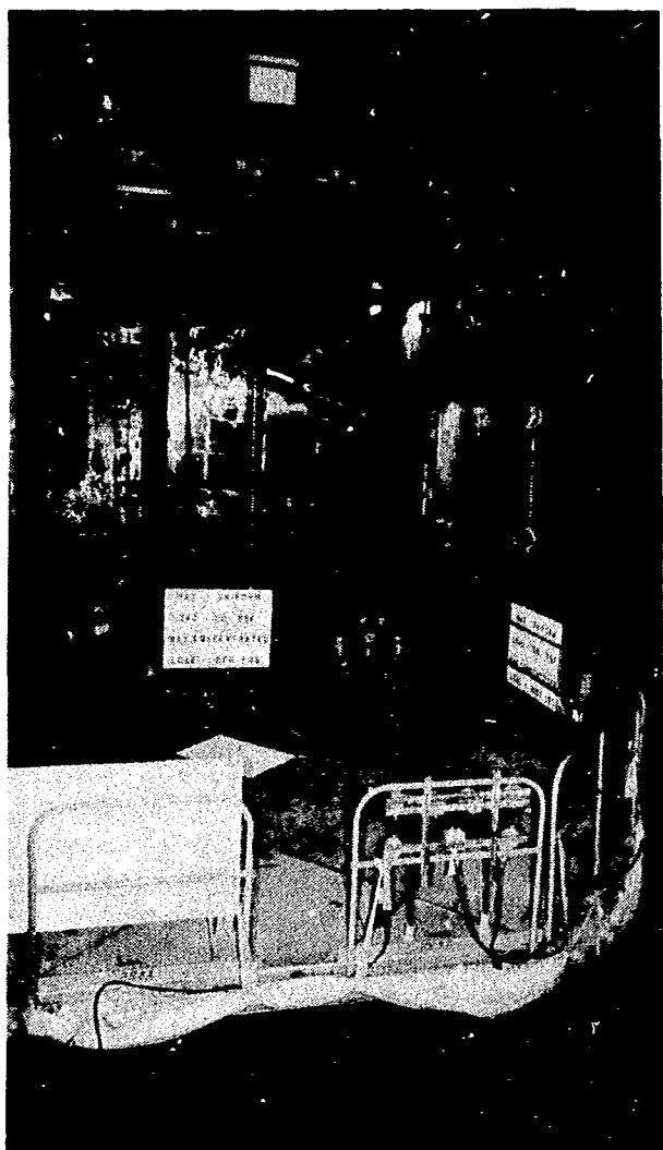
Figure 23. IIF platform, removable lead deck plates, and plenum misting system I-beam and vertical pipe.
